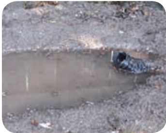
UNWANTED PONDING WITH CORRUGATED PIPE
