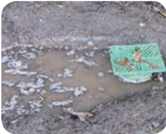
PONDING WITH CONVENTIONAL DROP INLET
